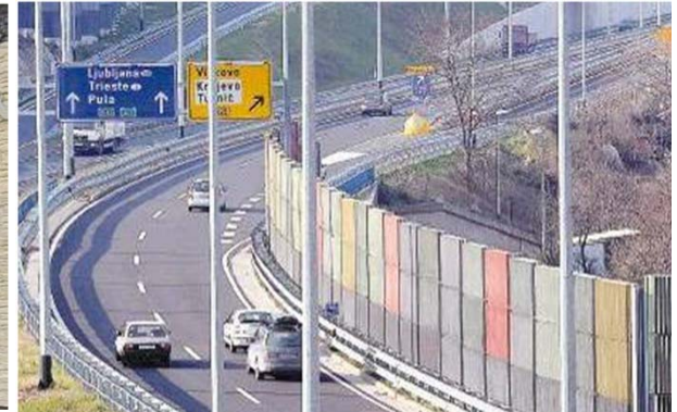
Bypass city of Rijeka (2009) aprox. 12.000 m 2
